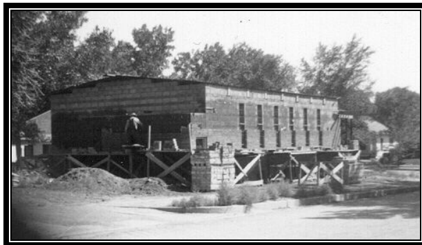
Church building under construction (spring/summer, 1953)
