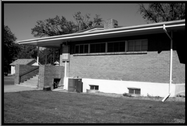
Church building seen from the south (fall, 2008)
